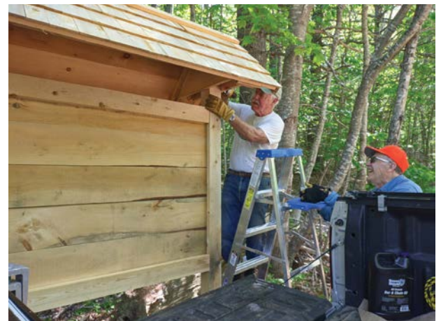
Volunteers Tom Earley and Bob Olfenbuttel install kiosk
