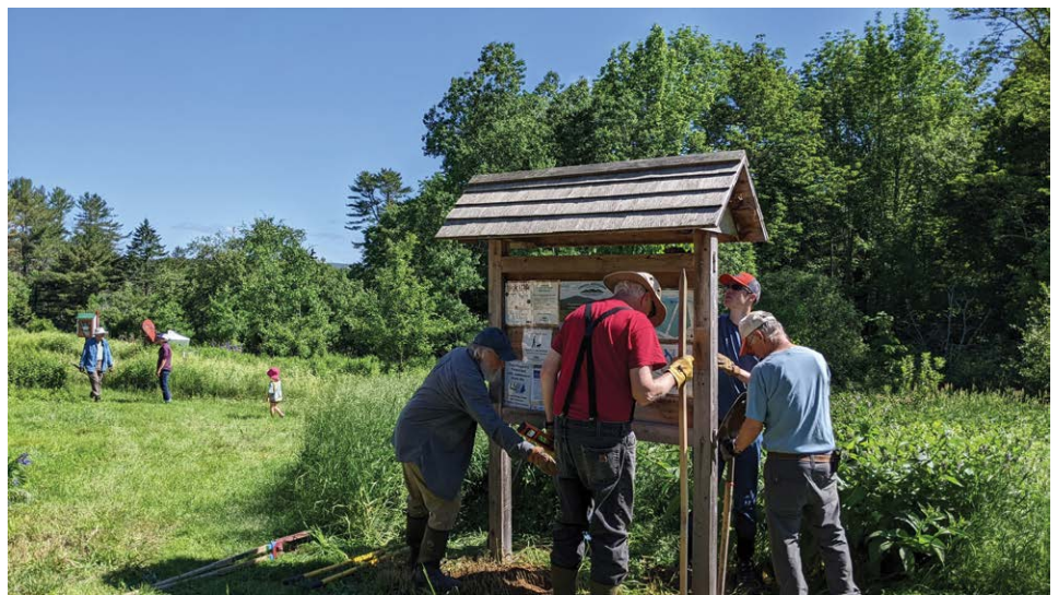
Installing kiosk at Head of Tide Preserve
