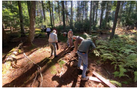
Removing bog bridge at Fernalds Neck Preserve
